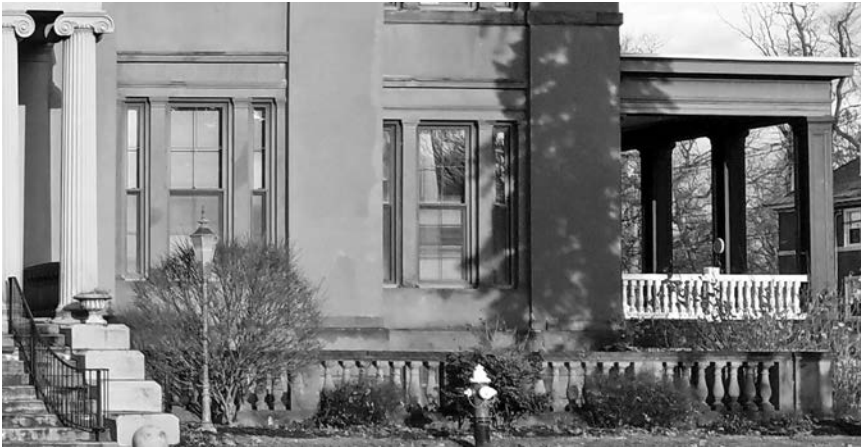
Detail of stone balustrades, c.2016. Photo by the author
