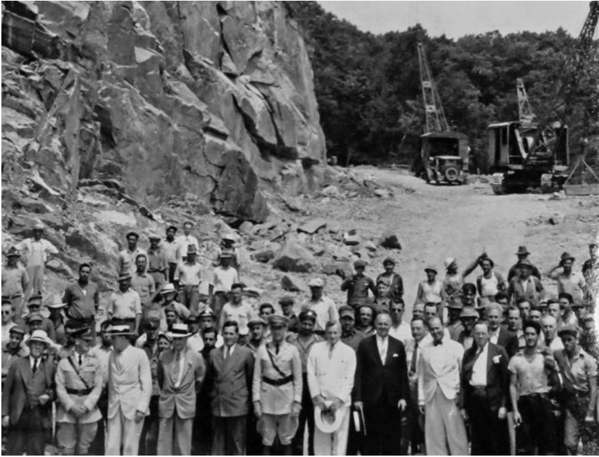
Devers (center, in uniform) on Storm King Mountain during the construction of Route 9W, c.1936
