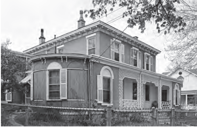
The Thornton Niven House c.1839-41, known as the Anthony House when inventoried as part of the Historic American Buildings Survey, at 201 Montgomery Street. Library of Congress
