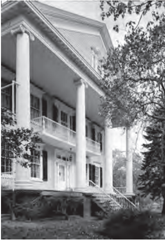
The David Crawford House, c.1830, 189 Montgomery Street, Historic American Buildings Survey, Library of Congress
